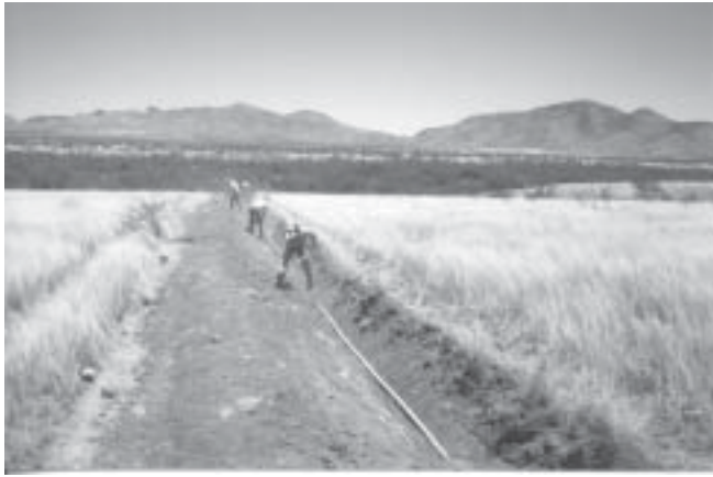
Figure 1 —Bedding water line across a loamy upland ecological site dominated by Lehmann lovegrass, spring 1982.
