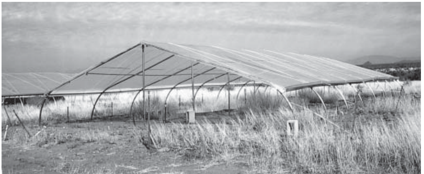
Figure 1 —Shelter (9 by 18 m, 4 m tall) on the Pleistocene site; open sides are 1.5 m off the ground. Tall grasses visible beneath the shelter are Heteropogon contortus . Note the cables attached to the shelter and steel fenceposts for greater wind stability, and polypropylene rope holding down the plastic cover.
